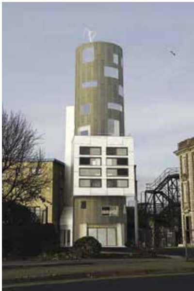
Tom Dixon Watertower House, London, SUSD
