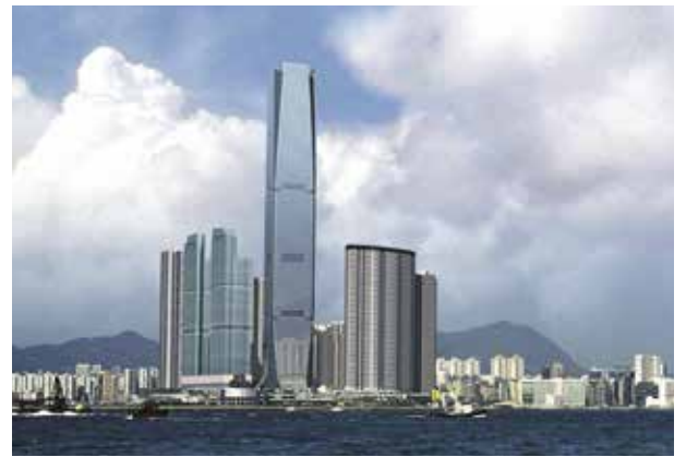
International Commerce Centre, Hong Kong, Kohn Pedersen Fox Associates
